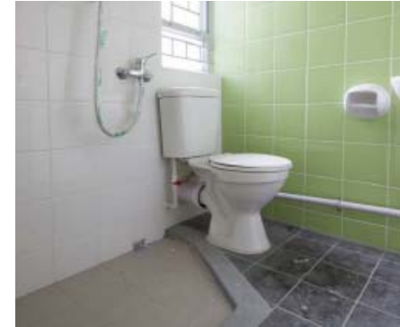
Basic fittings and provisions in toilets
