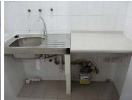
"High Level" suitable for built-in hob by cutting an opening to the polymer resin worktop (855mm from F.F.L)
