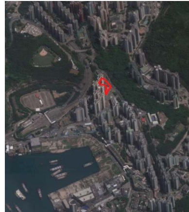
Eastern Harbour Crossing Site Phase 7 (~500 Flats)
