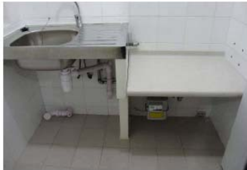
"Low Level" suitable for Gas Cooker (595mm from F.F.L)
