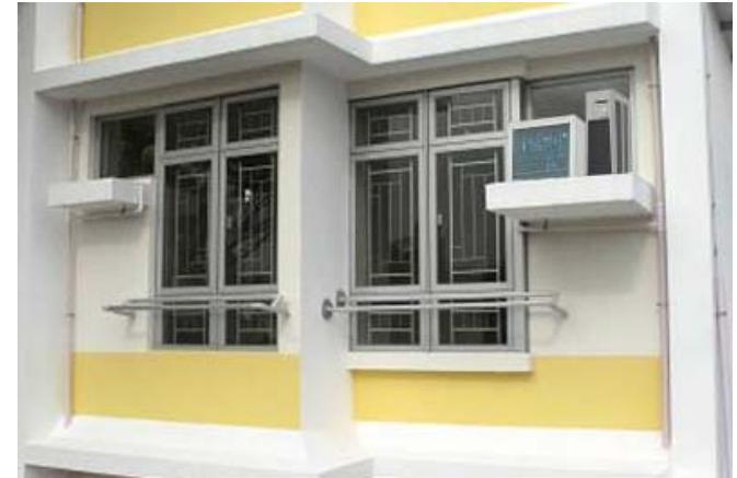
Extensive use of multi-layer acrylic paint on fair-faced concrete instead of wall tiles
