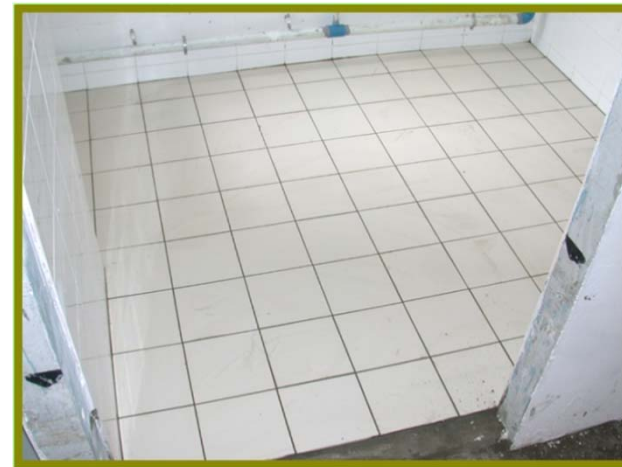
Homogeneous floor tiles to kitchens
