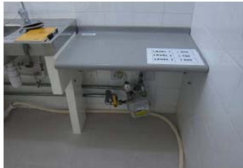
"Middle Level" suitable for Induction Cooker (755mm from F.F.L)
