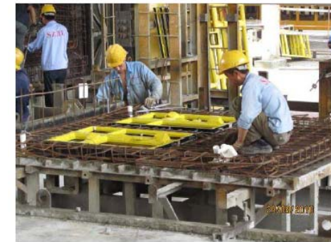
Precast Façade - Rebar and window fixing
