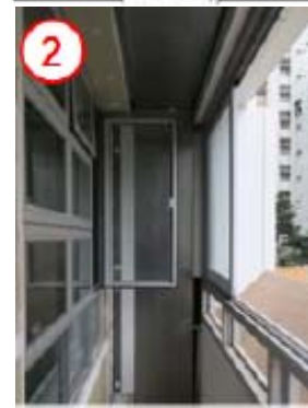
2 nd Generation Acoustic Balcony (2016) (- 6 to 10 dB(A)) Better Noise Attenuation Better Ventilation
